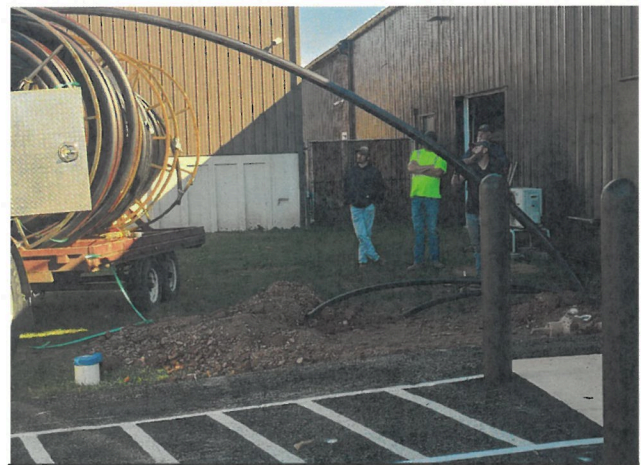
Boring Process Underway to move the township building's overhead wires underground.
