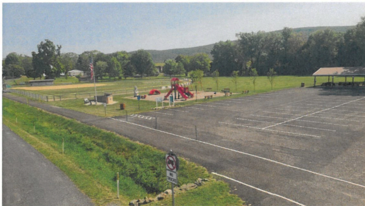
Loyalton Park Parking Lot was lined to make parking easier
