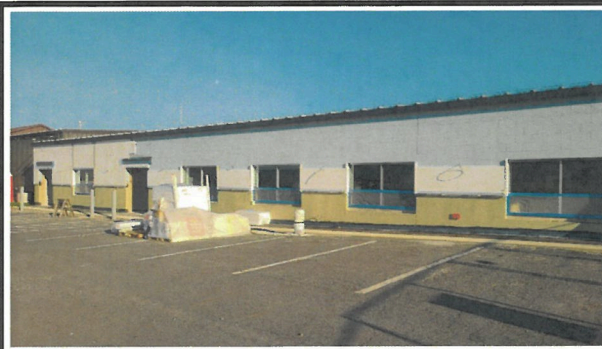
Left: Outside of building with outside finish started and windows installed.
