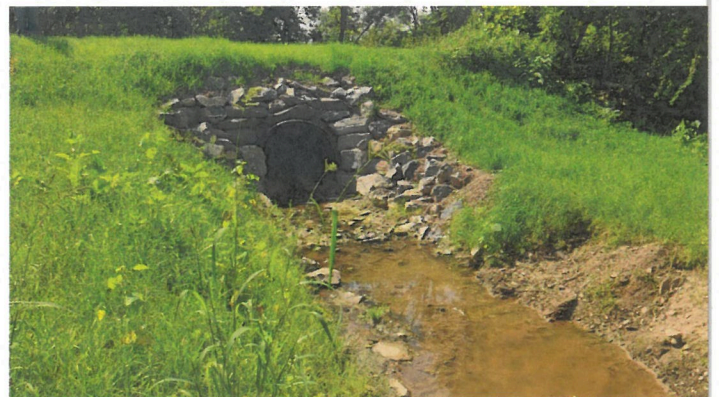
Pipe was installed on Bechtel Road.
