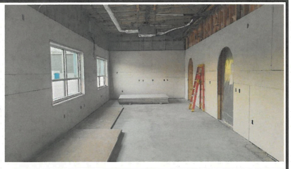
Right: Inside of what will be the new offices for the District Court. HVAC, wiring and drywalling completed.
