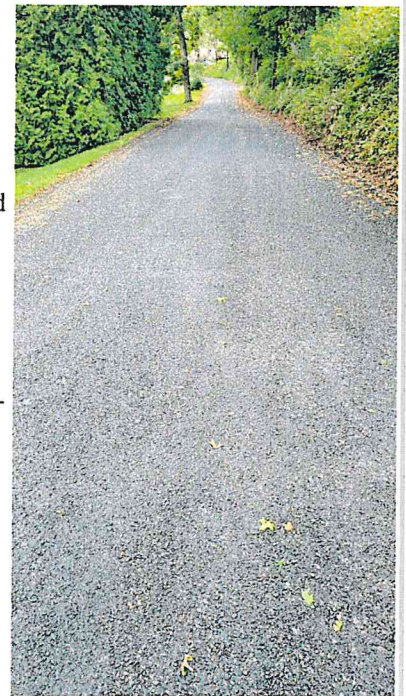
Lenker Road had the berms cut, spot patching and the roadway Seal Coated and Fog Sealed
