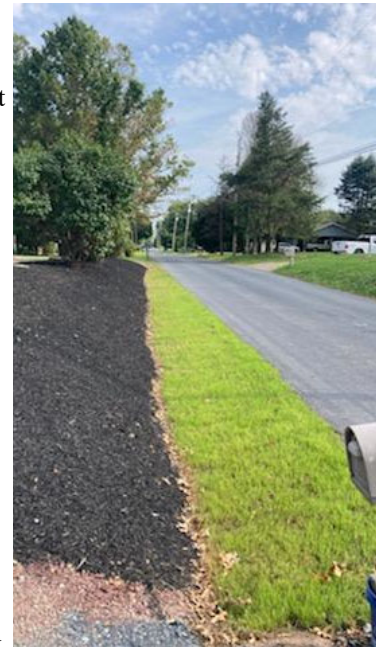
A grass berm was added on North Stone Road to stop the erosion that was occurring along the edge of the Cartway.
