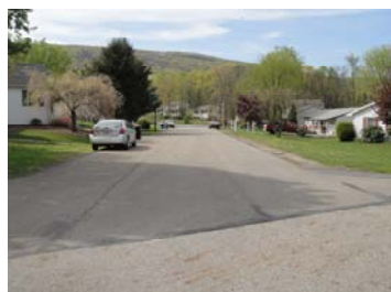
This part of Steve’s Lane to be widen & paved this year.
