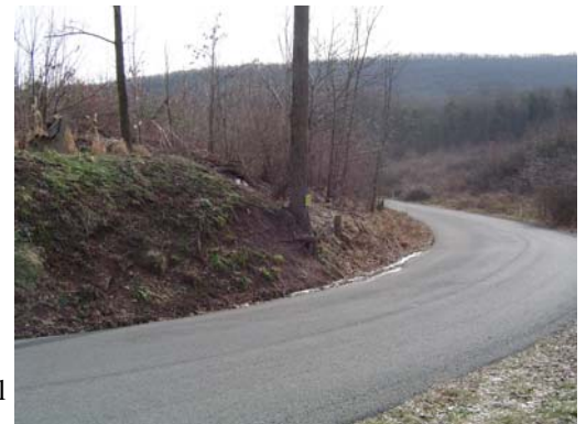
Part of Mohr Road will be widened to match the rest of the road.
