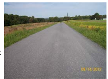
Henninger Road was widened, leveled & seal coated. Wider berms were added.
