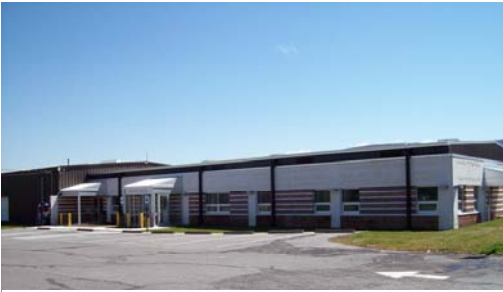
Washington Township Municipal Building
